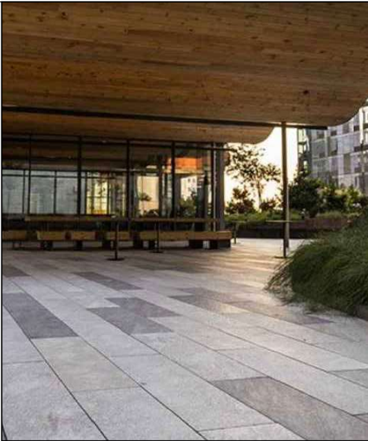
3. PORCELAIN TILE PAVING ON PODIUM (MATCH INTERIOR TILE)
